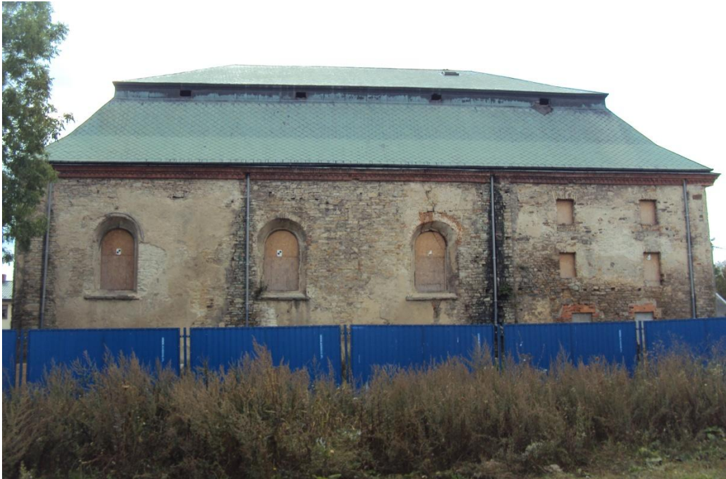
1. The deteriorated synagogue in 2013. Source: Private collection.
