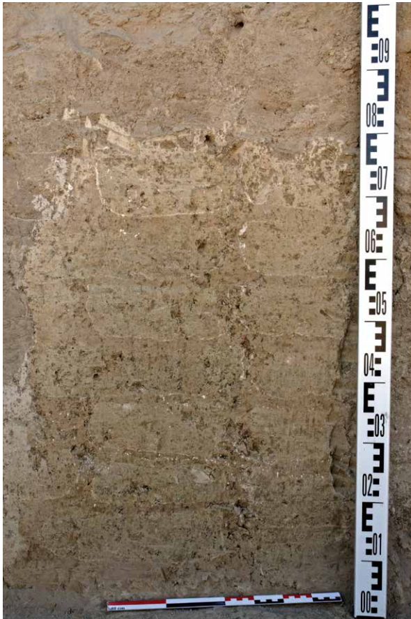
Fig. 4.6. Detail of the eastern profile of wall 290, with the thin white coating of the bricks and the reddish mortar visible.
