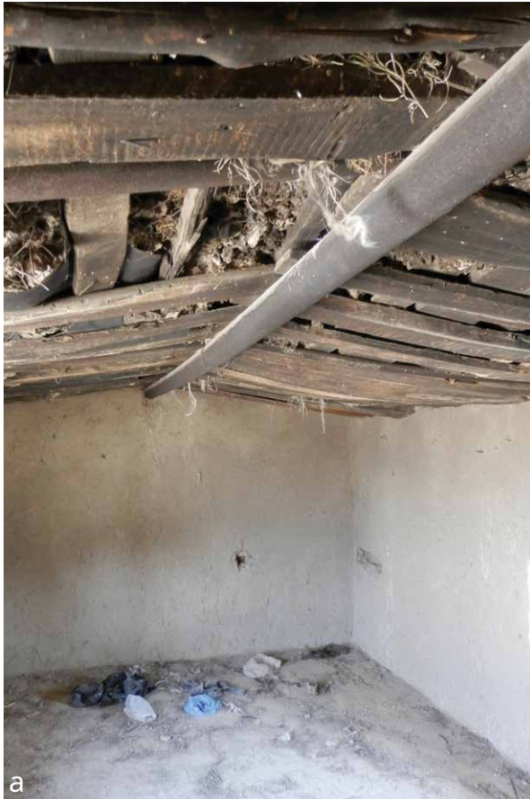
Fig. 5.15. Roof structure in a shepherd's hut in the vicinity of Meana. A: view of ceiling; B: the hut; C: detail of the ceiling: compact mud fill with vegetal material inside an iron mesh with a thin asphalt coating.
