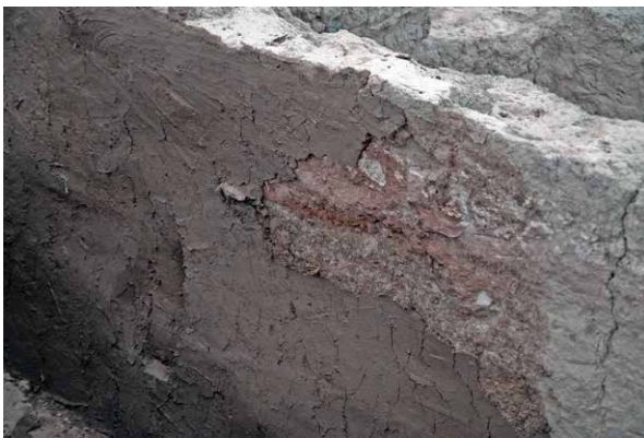
Fig. 2.8. Wall covered with mud plaster prior to backfilling.
