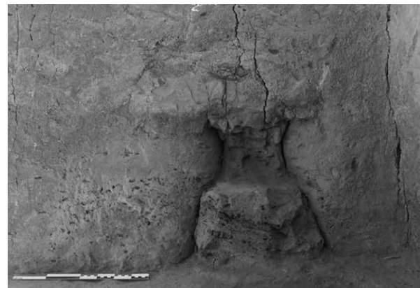
Fig. 5.3. Entrance in wall D467.
