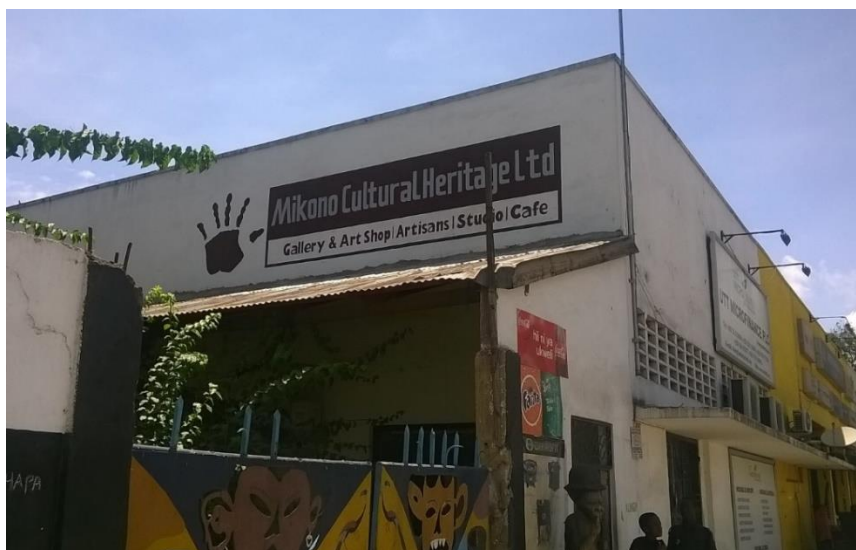
Fig.133 A recent photo of the National Arts of Tanzania or HANDICO Building, currently the Mikono Cultural Heritage Ltd, in the Chang'ombe area of Dsm (Photograph by researcher, September 2015)
