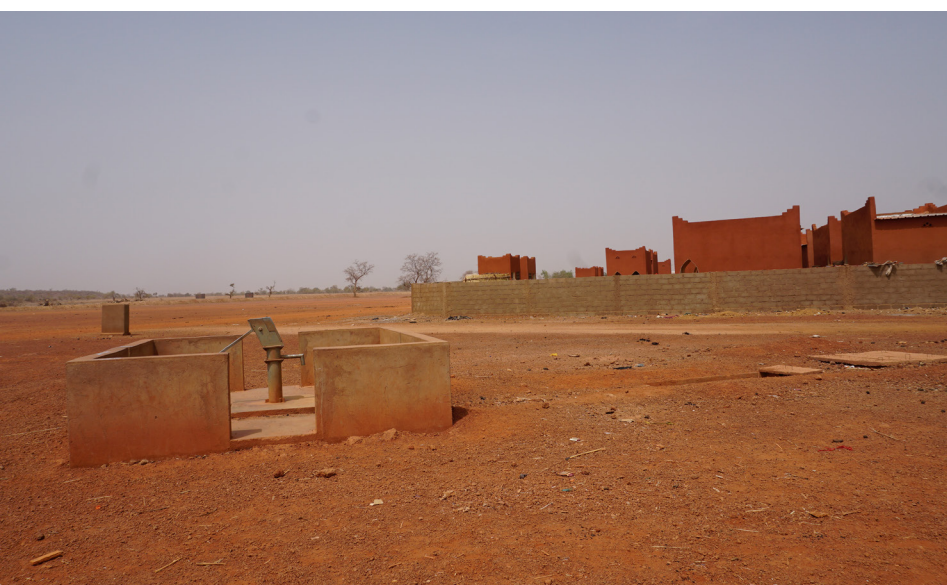
Non-functioning well in the newly constructed Bouly village (Photo: Merle Groneweg, 2017)
