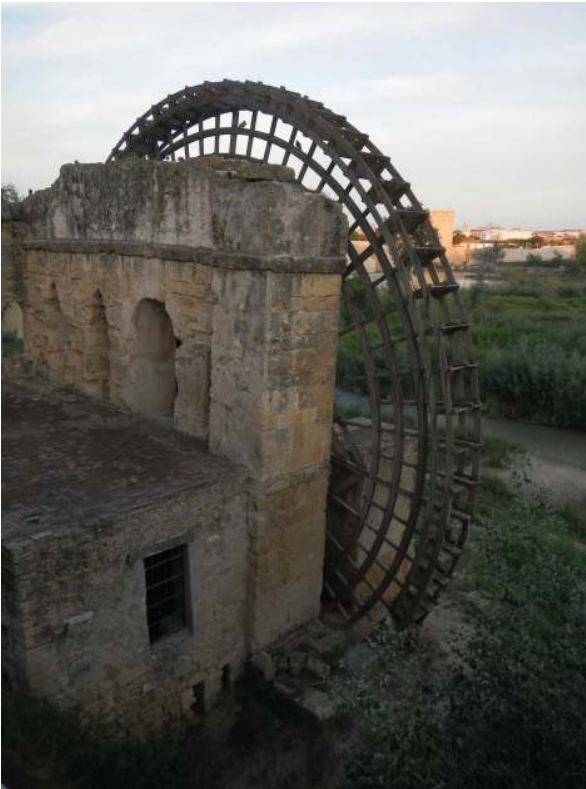
Fig. 6 This typical example of a noria (water-wheel) was reconstructed on the Guadalquivir River in Córdoba. Possibly, it was originally built by the Romans and modified in medieval times to provide water for Alcázar de los Reyes Cristianos (a medieval castle) for gardening and for milling grain. This noria was powered by the river.
