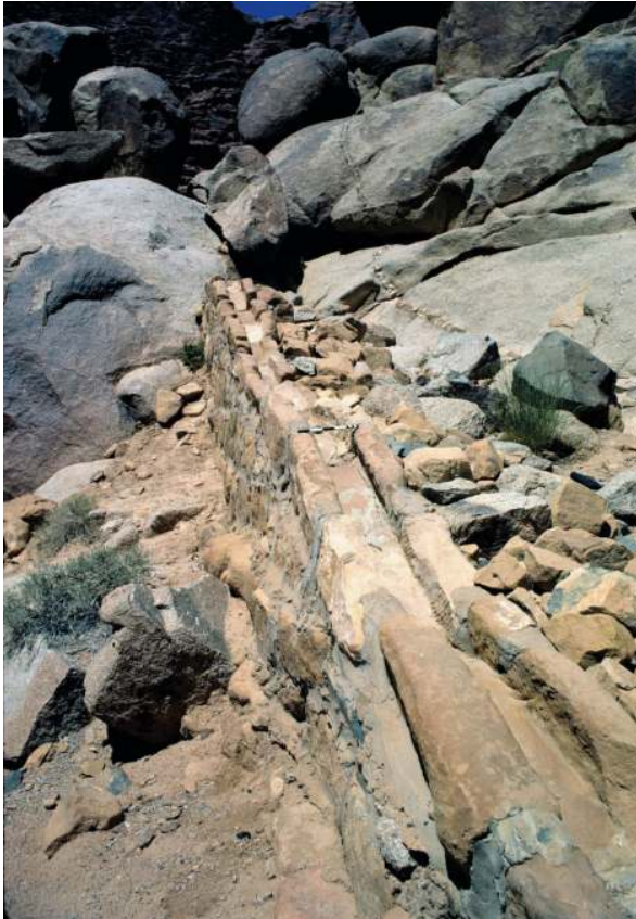
Fig. 14 Aqueduct channel, Ramm.
