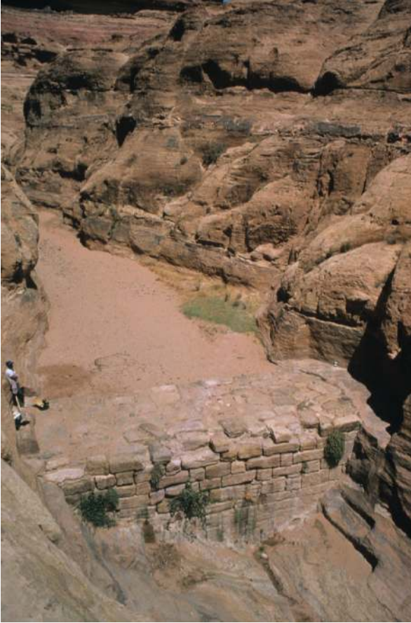
Fig. 13 Nabataean dam, Hawara.
