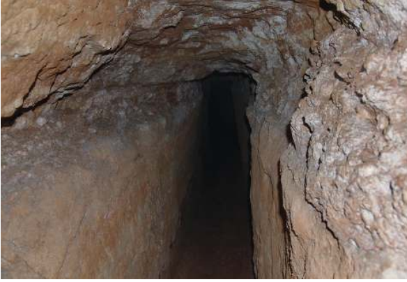
Fig. 12 The adit at Bureta is some 100 m long, 2 m high and c.9 m wide.
