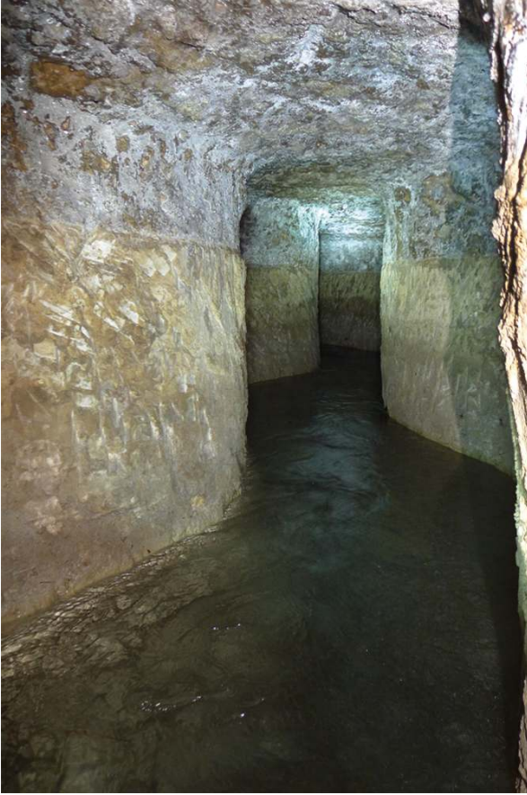
Fig. 7 Track of the Aqueduct in the Hyblaean Mountains.
