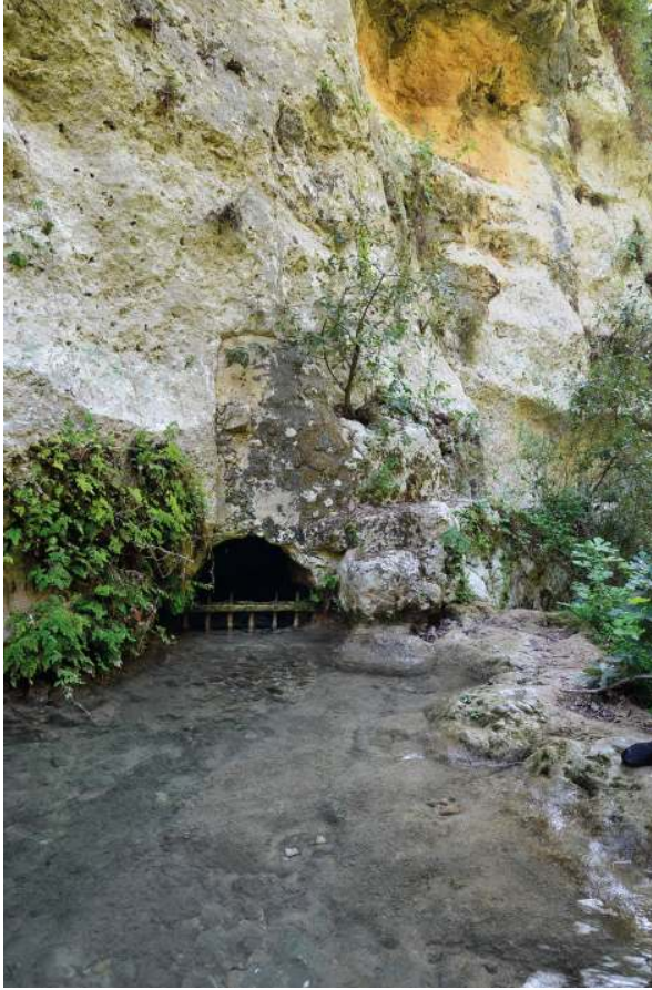
Fig. 4 The Calcinara water intake.
