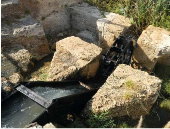
Fig. 9 Undershot wheel installation of a reconstructed Byzantine water mill at the river Nahal Tananim. This structure is a good example of ancient water-mills that still function.
