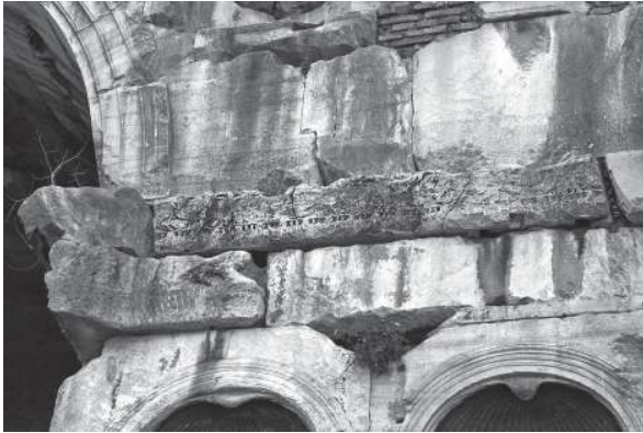
Fig. 2 Arch of Janus: reused decorated frieze set in inside the masonry and not destined to be seen.
