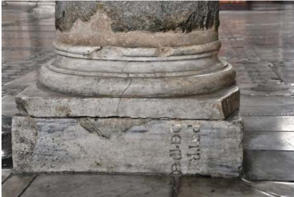
Fig. 30 S. Maria in Aracoeli: base from the late second century with a pedestal block with a mediaeval inscription.
