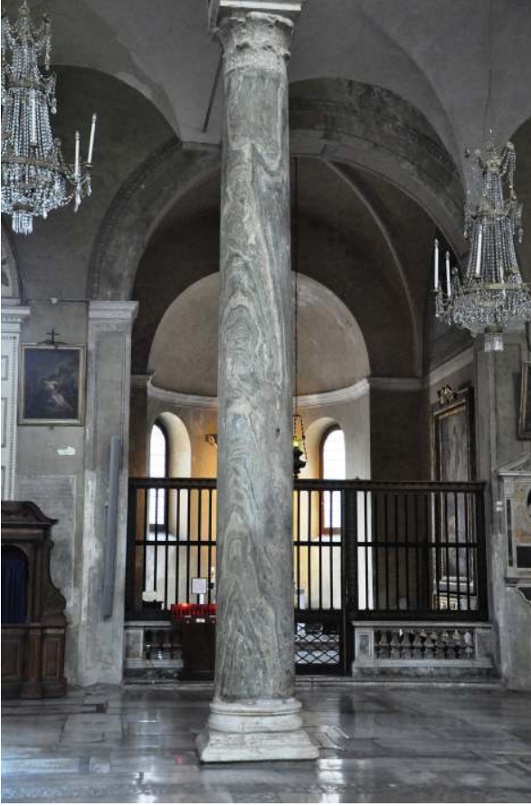
Fig. 27 S. Maria in Aracoeli: column shaft in cipollino marble with a Constantinopolitan Corinthian capital (late fourth – fifth century).
