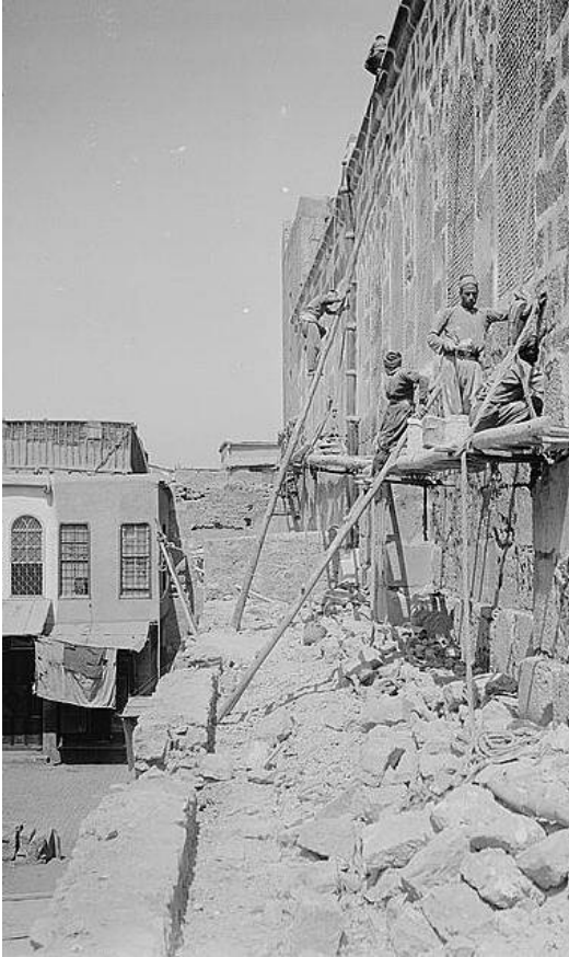
Abb. 20: Restaurierung der Umayyadenmoschee [399], ca. 1895 (Library of Congress)
