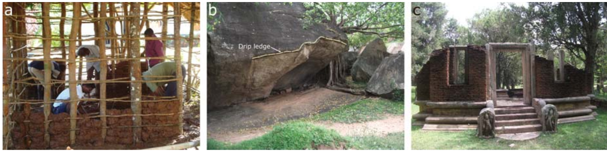
Figure 2.1.: Landmarks of the architectural history of Sri Lanka. (a) Constructing a wattle and daub house, following the primitive methods (Kebithigollewa Buddhist temple in 2010) (b) Prepared natural rock shelter. The drip ledge can be seen over the roof portal (Vessagiriya monastery 2014). (c) Conventional monastic architecture: constructed using stone and brick materials (Abayagiriya monastery 2014) (Photographs taken by Wagalawatta.)
