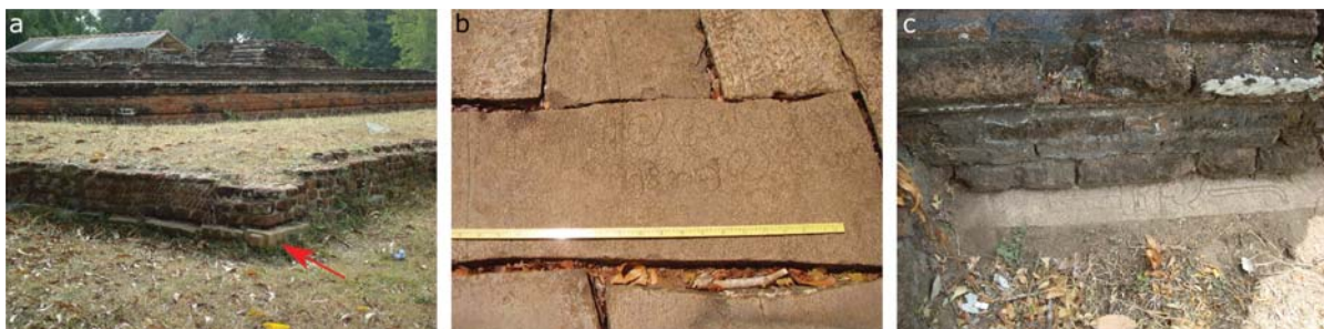
Figure 2.2.: Evidence about re-used building materials; (a) The red arrowhead points to a foundation slab in the Vijayabahu palace (10 th century CE) (Citadel). It is a fragment of a former door or window frame. (b) Fragment of a 'slab of inscription' used as a paving stone (Asokaramaya monastery) and (c) a former 'pillar Inscription' used as a foundation slab (temple of the tooth relic in the Citadel) (Photographs taken by Wagalawatta.)
