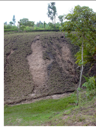
Fig. 33: Landslide on Steep Slope
