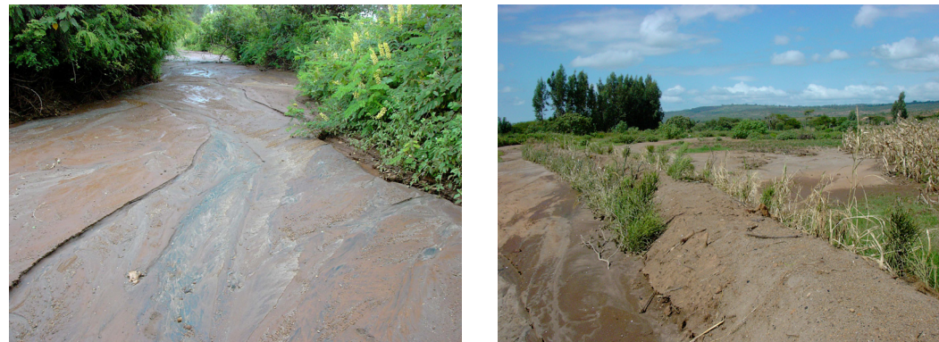
Fig. 48: Sedimentation in a Channel and on the Alluvium
