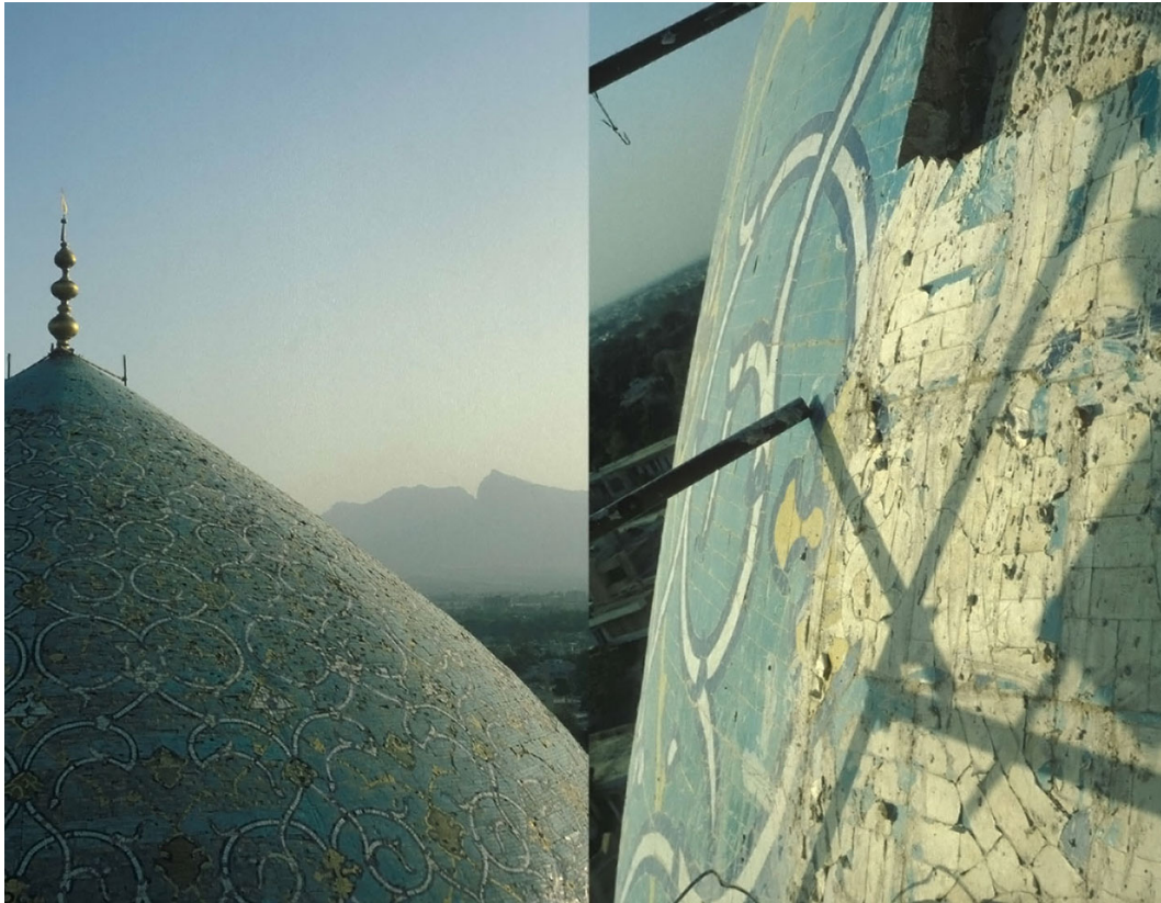
Fig. 13 | Masjed-e Shah in Isfahan (Iran), dome of the mosque. Left: the historical tile mosaic. Right: its skillful modern replacement.
