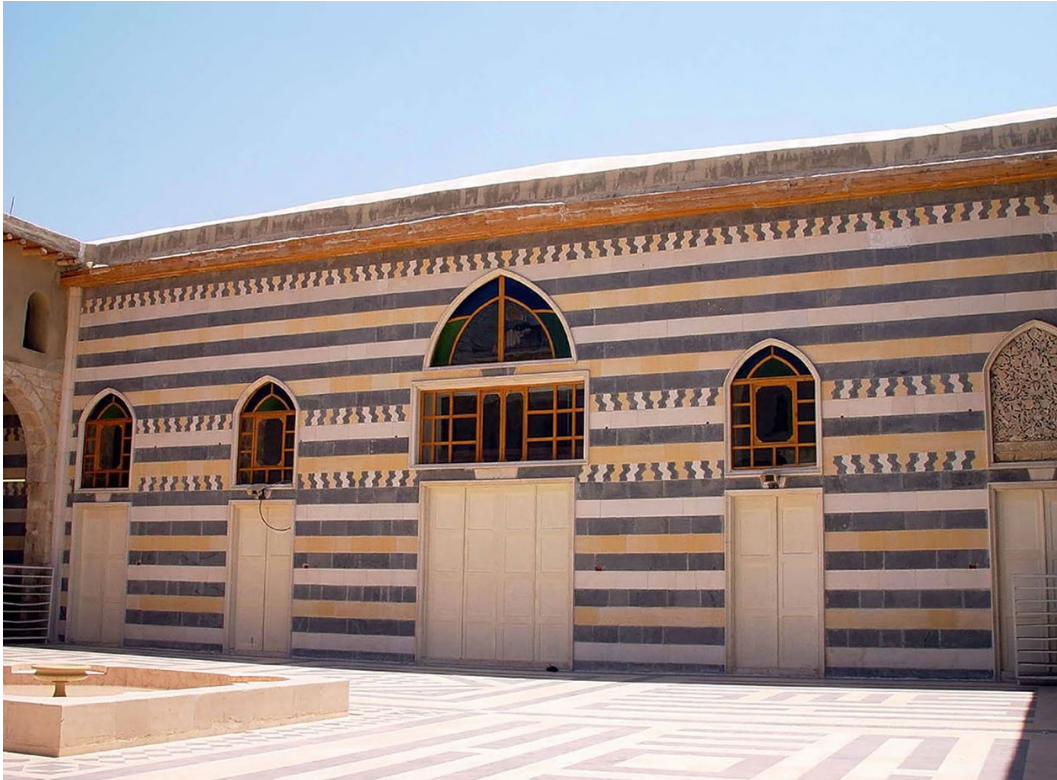
Fig. 14 | Hanabila Mosque in Damascus / al-Salihiyya (Syria), cladding of a historical mosque from the 12th c. in a free modern interpretation of a much later style, combined with the cleaning of all historical material inside the courtyard.
