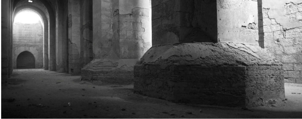
Fig. 8 | The “large cistern” in Resafa, Syria. It was filled by channeling periodical floods from a wadi west of the city into the cisterns and had a capacity of \sim 18,000 \text{ m}^3 .
