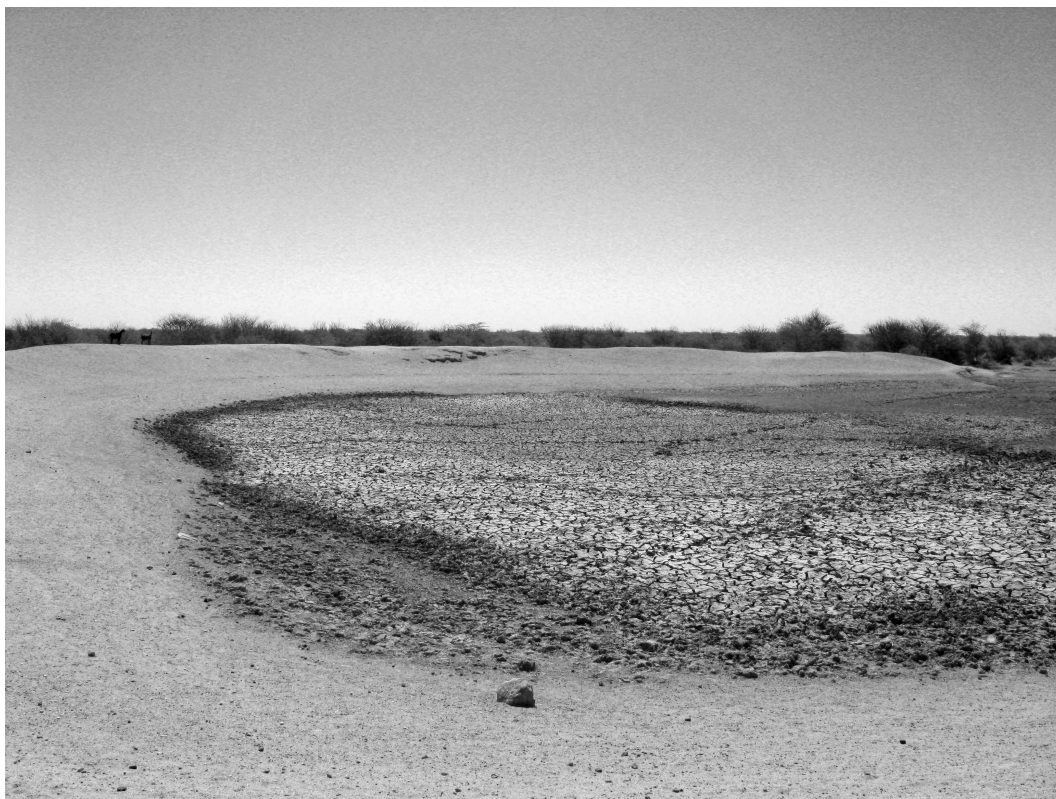
Fig. 5 | A desiccated hafir in the Sudan. Note the goats standing on the embankment to the left of the photo for scale. The hafir is filled from the right by a wadi.
